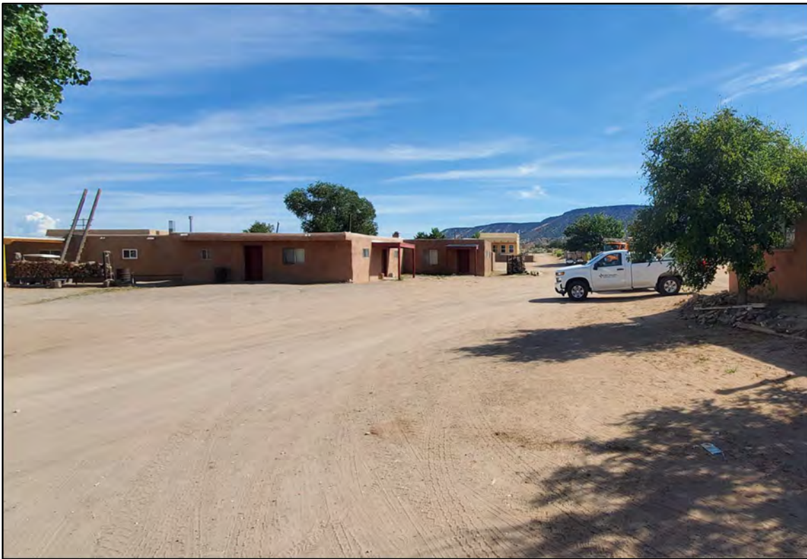
General Site Conditions, View Toward the NE from the Vicinity of B-2
